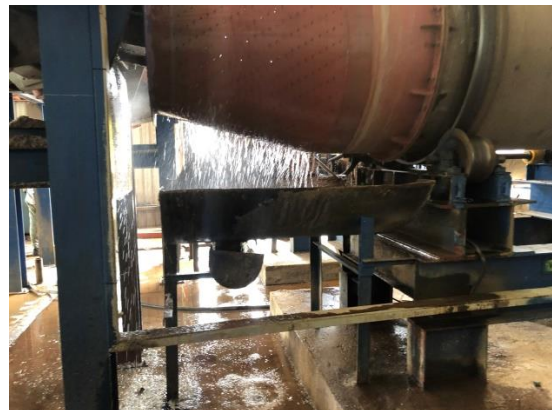
Cullet washing plant.
